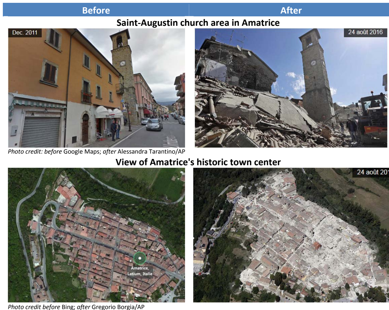
FIGURE 5: AMATRICE: BEFORE AND AFTER THE EARTHQUAKE 3
